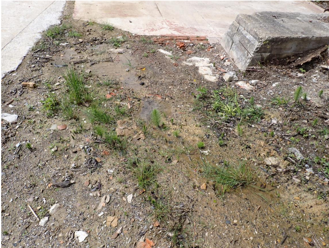
Photograph 9. Area of impeded water within the centre of the northern section of the site.
