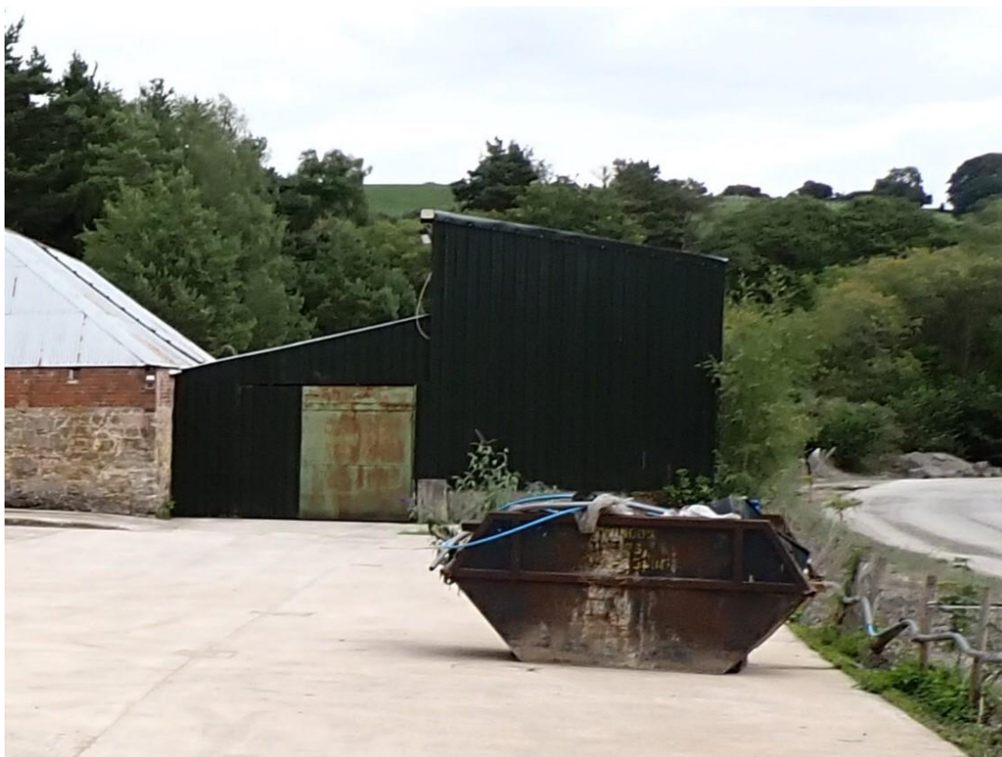
Photograph 11. The western aspect of Building 1.
