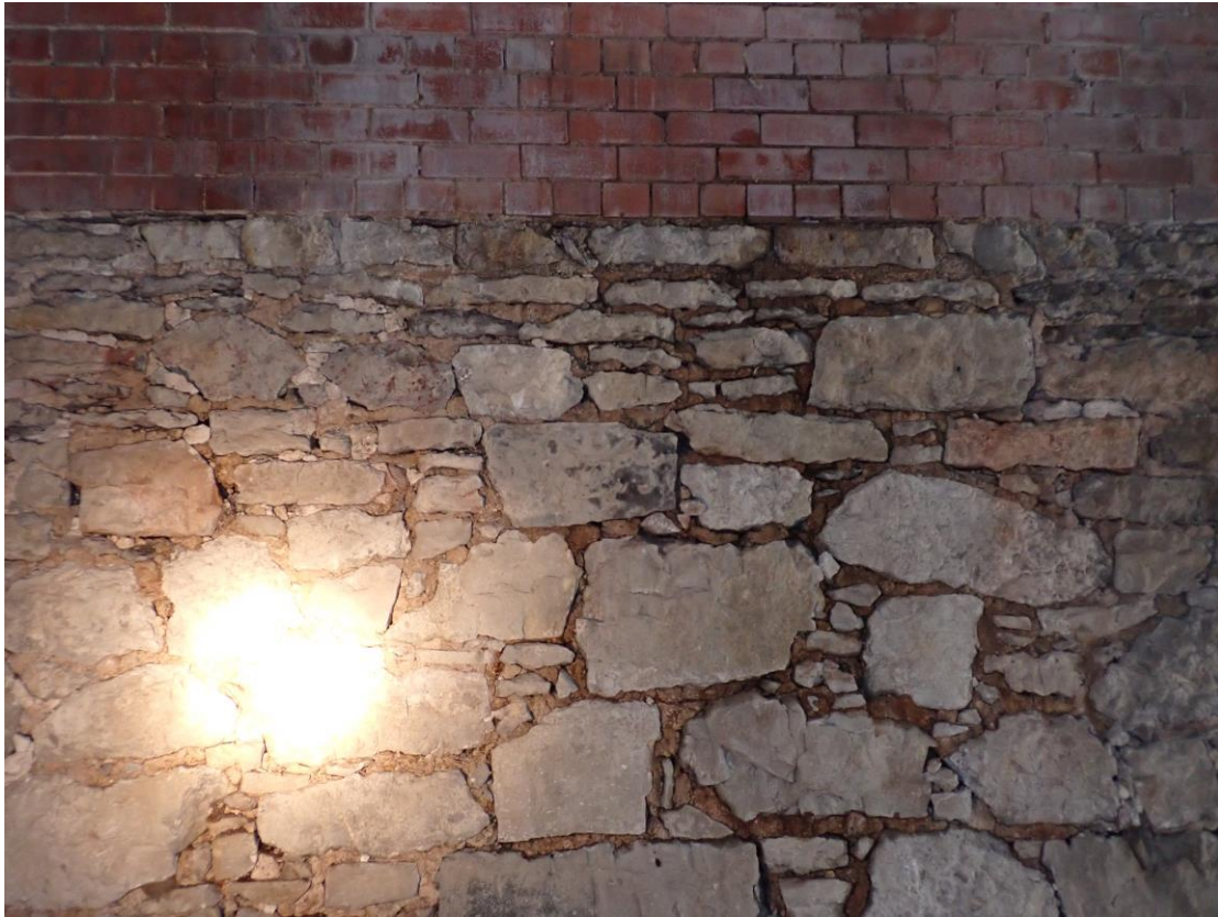
Photograph 15. Cavities within the external walls of Building 2.
