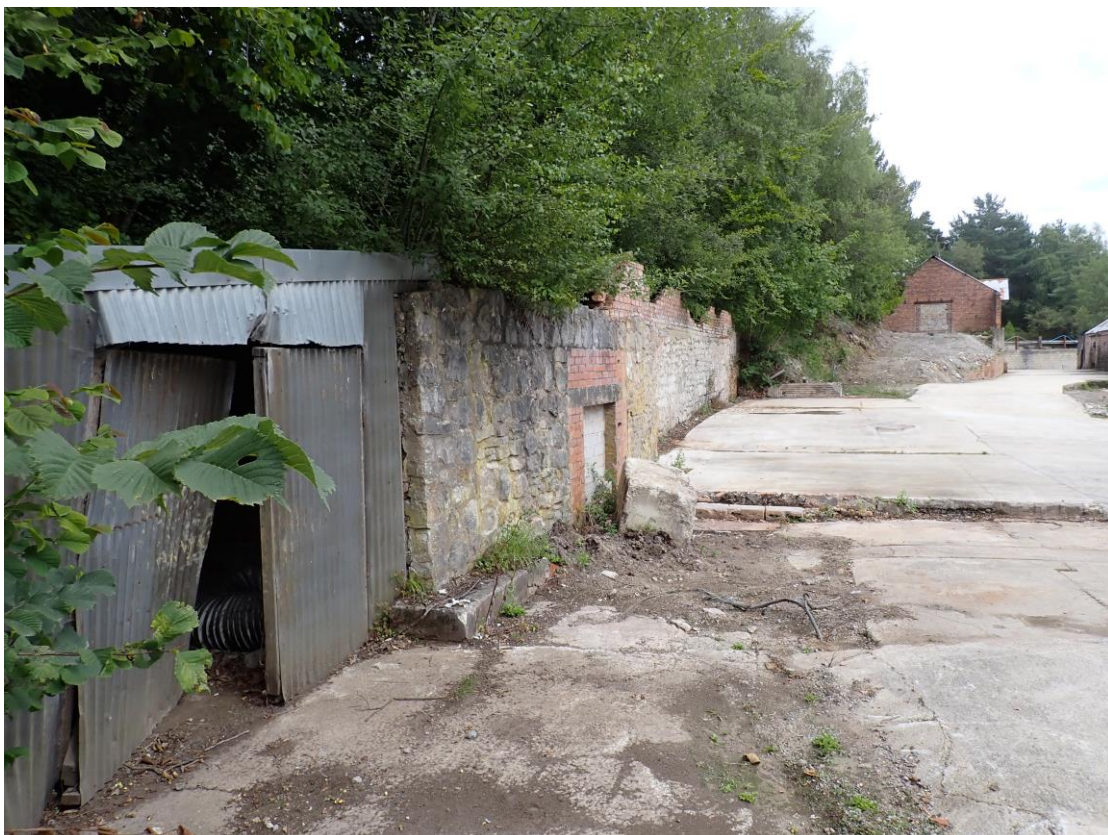
Photograph 10. A stone and brick wall along the northern boundary.
