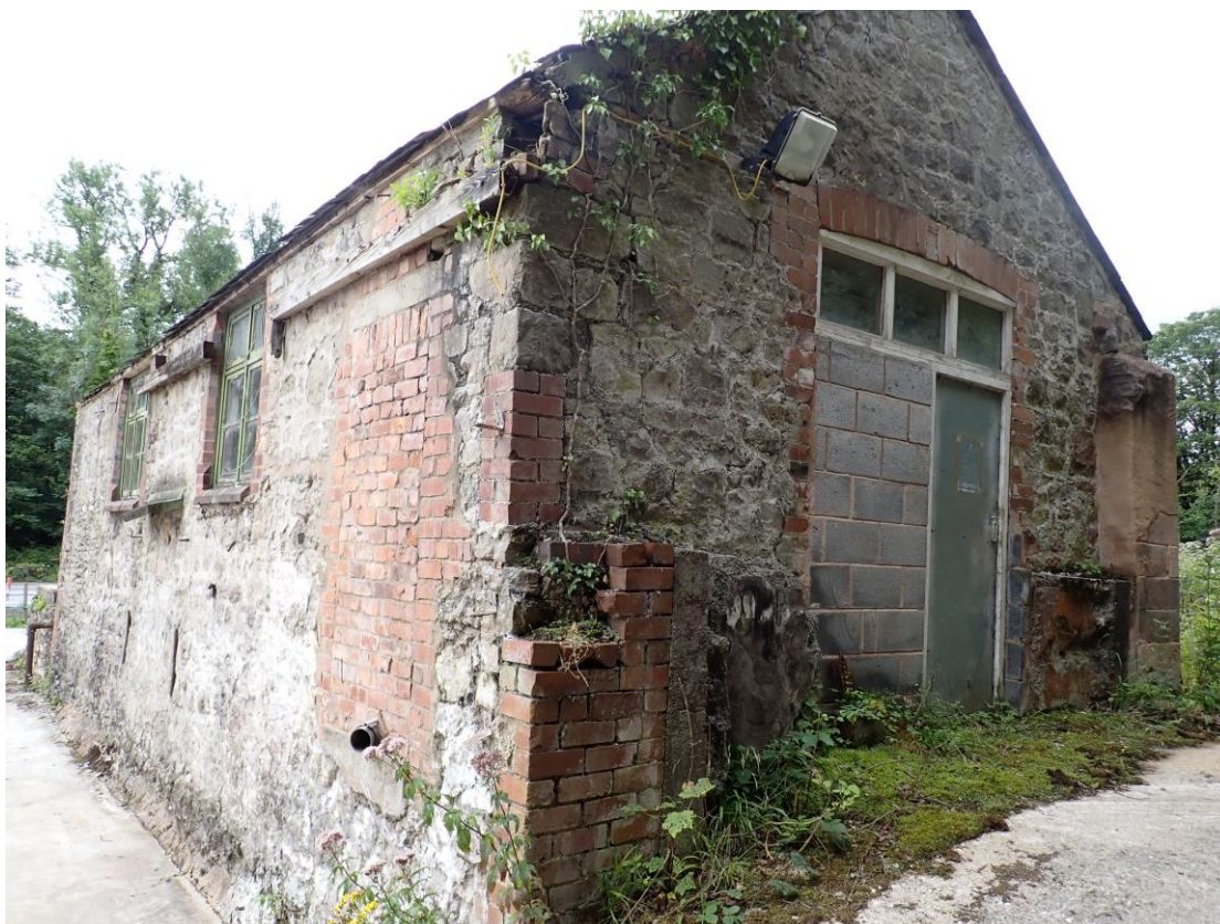
Photograph 13. The northern aspect of Building 3.
