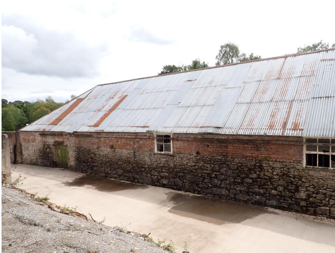
Photograph 12. The northern aspect of Building 2.
